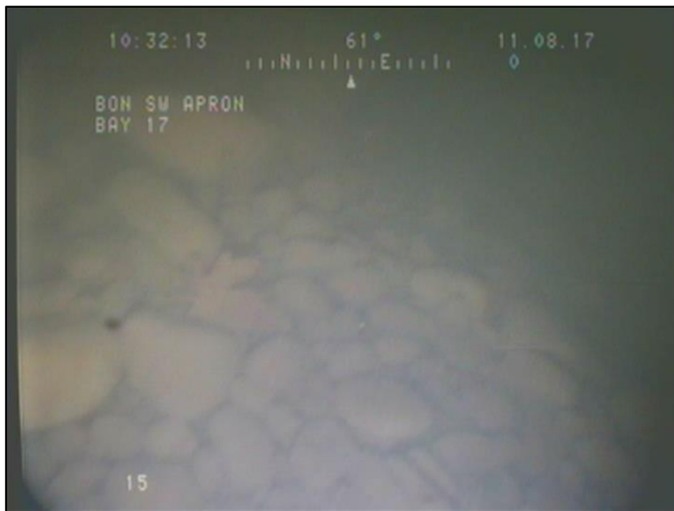
Figure 4 Rock pile in SB 17 on the shallower upstream edge.
