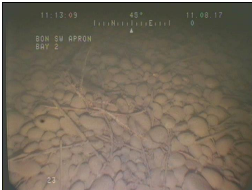
Figure 14 Rock debris and pieces of rebar found in SB 2.
