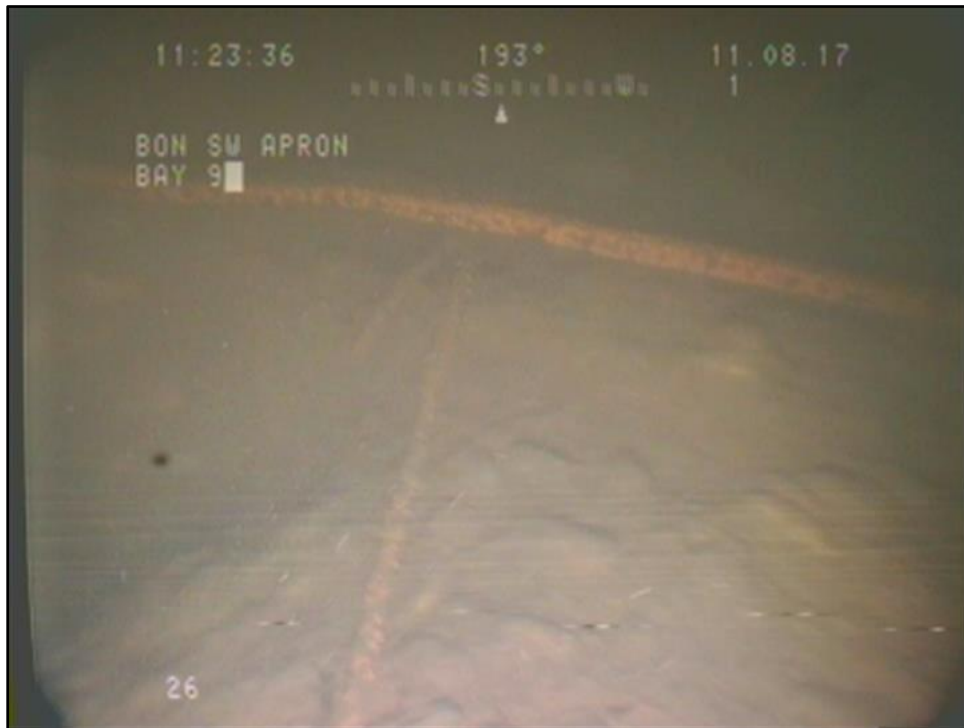
Figure 9 Significant erosion found between baffle rows at SB 9.
